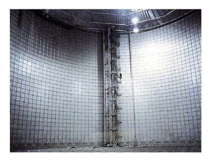
Membrane Tank - A tank that uses a thin metallic liner as the inner tank. Unlike a conventional metal tank (which is self-supporting), a membrane cannot support its own weight and must be supported by other means.
